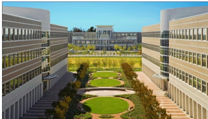
Greenville Hospital Medical Office Portfolio: Patewood Campus, Greenville, SC Acquired September 2009
